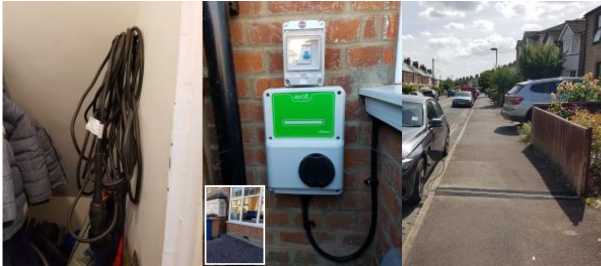
Figure 7. These images of the APT home charger and cable channel highlight the four main parts of the system, namely an extended cable, the wall box charge point and RCD (residual current device) box and the cable channel. Depending on the location of the wall box on the house, the length of the trailing cable and how close the user is able to park to the end of the cable channel this can also be a largely inconspicuous way of charging. Pictures taken by: B. J. Doody.
