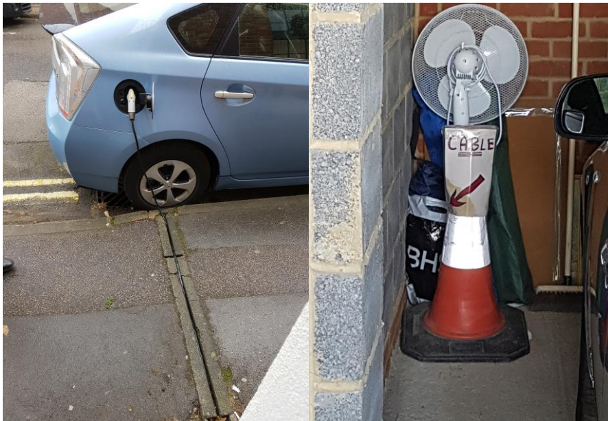
Figure 2. Two examples of how trial participants used temporary and informal measures such as road cones and rain drains to reduce the chances of someone tripping on the cable while charging their electric vehicle. Picture taken by: B. J. Doody.
