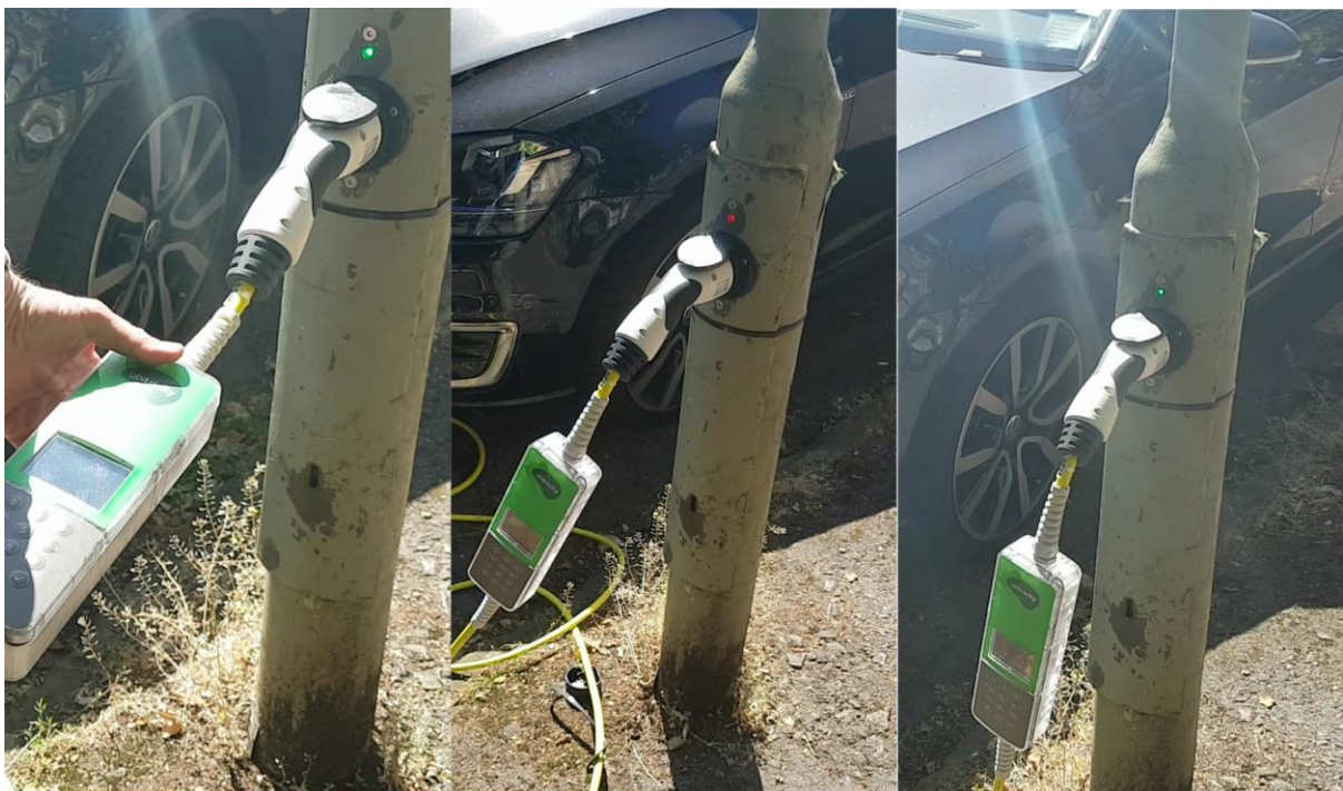
Figure 6. Three video stills capturing how Daniel's car after successfully plugging into an Ubitricity lamppost installation (left video still) stopped working even though his battery was not at full capacity (centre video still) and then resumed after being unplugged and re-plugged in (right video still). Video recorded by: B. J. Doody.
